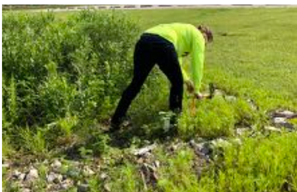
SGRWA working on maintenance at Justice Center rain garden.
